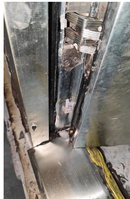
Photo 21 - The bottom right corner of doorset after medium temperature test
