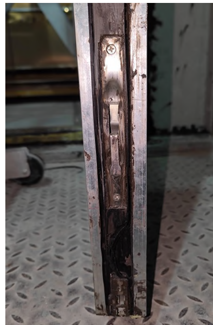
Photo 25 - The position of flush bolt after medium temperature test
