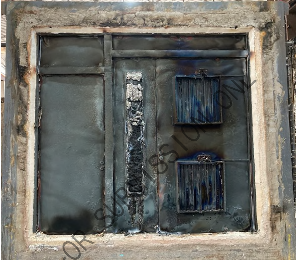
Photo 7 - The unexposed surface of the specimen after the test
