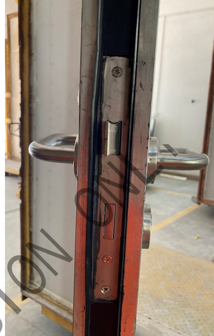
Photo 8 - The position of latch after medium temperature test
