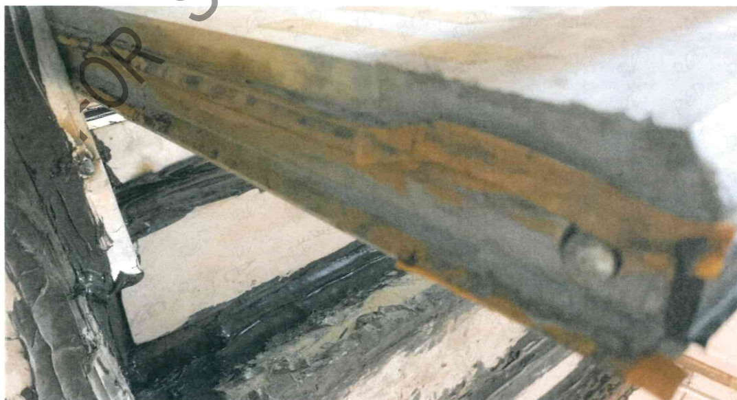
Photo 8: Fire and smoke seals arrangement at the bottom edge of both door leaves
