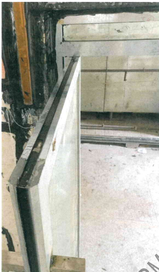
Photo 7: Fire and smoke seals at the top edge of the door leaf
