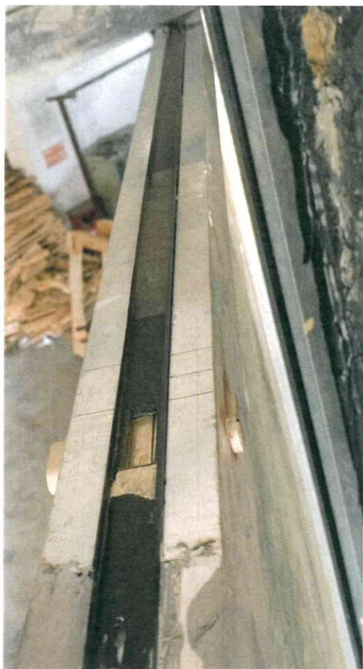
Photo 7: Fire and smoke seal at the top edge of the door leaf
