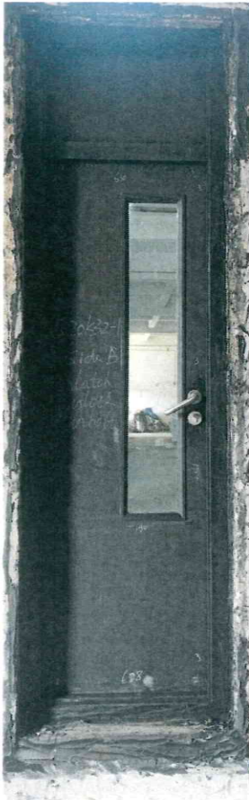
Photo 1: Exposed face of Doorset before the test.
