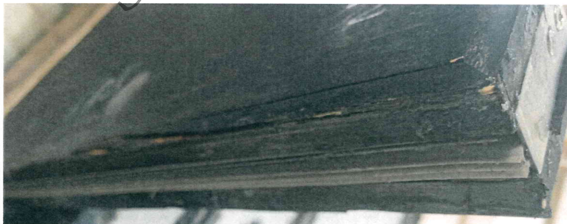
Photo 10: The automatic drop seal at the bottom edge of door leaf
