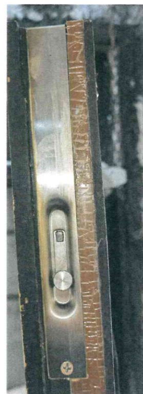
Photo 10: No smoke seal at the meeting edge of the PASSIVE door leaves
