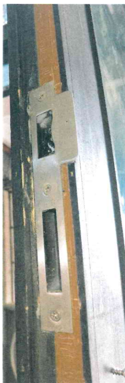
Photo 10: No smoke seal at the meeting edge of the PASSIVE door leaves
