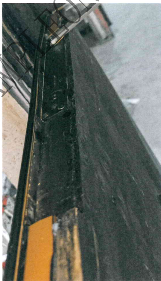
Photo 8: Fire and smoke seal arrangement at the top edge of door leaf.
