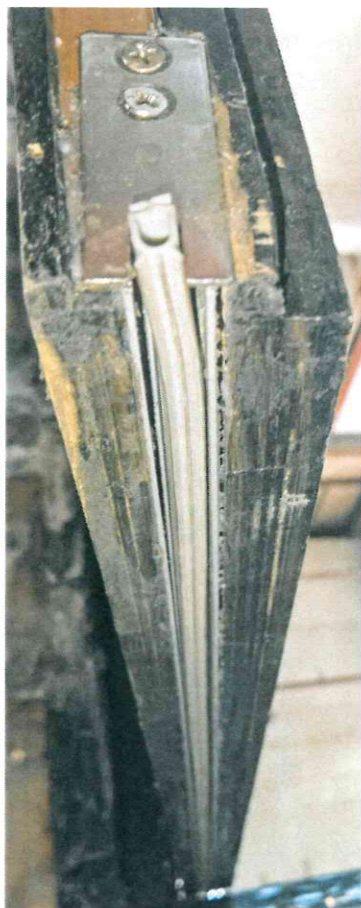
Photo 11: The automatic drop seal at the bottom edge of leaf.
