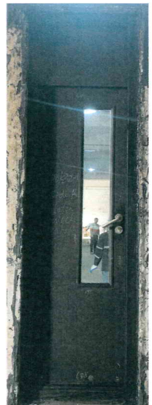
Photo 2: Exposed face of Doorset after the test.
