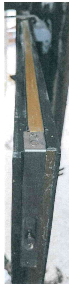
Photo 8: Fire and smoke seal arrangement at the top edge of door leaf.
